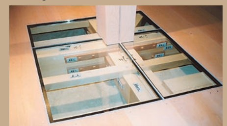
▶ Framework under the floor and the inside of walls
